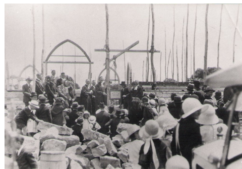
Laying of the foundation stone
